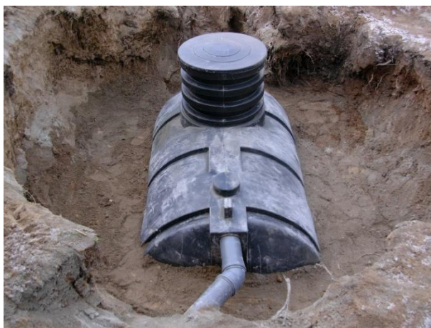
Figure 1. Septic tank assembly
