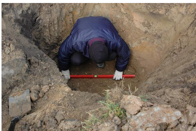
Figure 5. Leveling the bottom of the excavation
