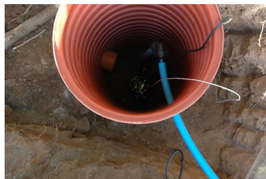
Figure 2. Pumping station in the excavation
