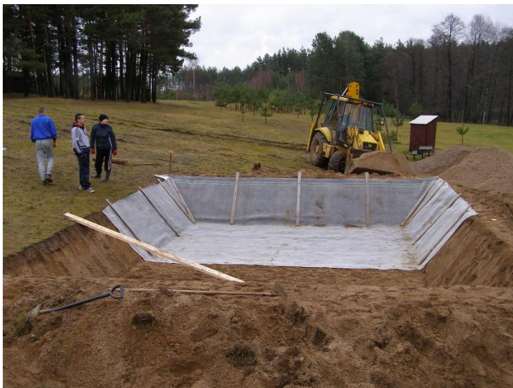
Figure 6. Implementation of the second filter layer - bentonite mat.
