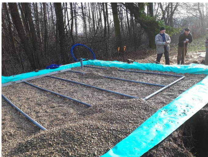
Figure 12. Infiltrating drainage in the backfill
