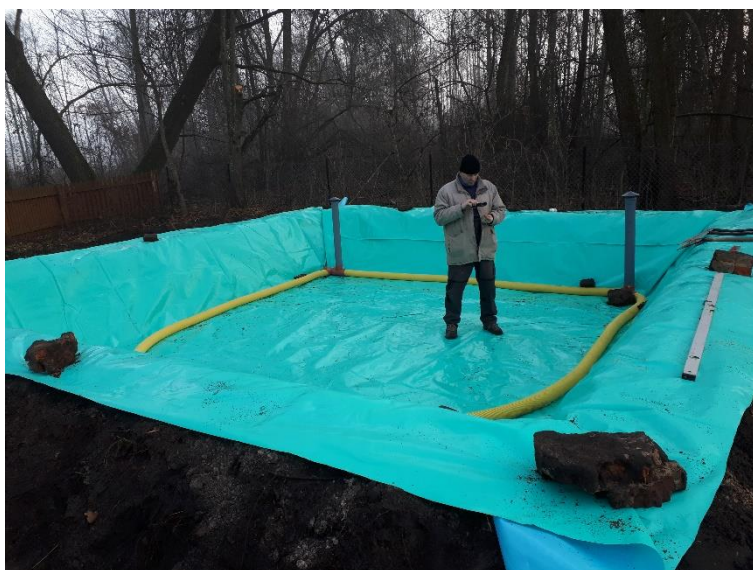
Figure 7. Collecting drainage
