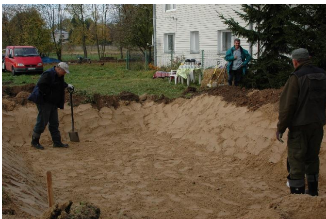
Figure 4. Making the first layer of the filter – sand for the film.
