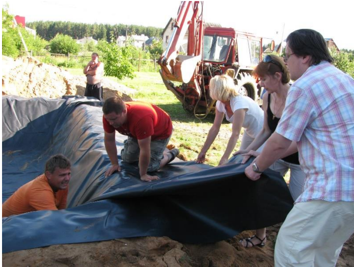
Figure 5. Spreading the second layer of the filter - foil
