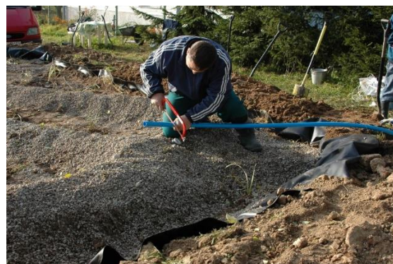
Figure 2. Connection of the settler tank to the infiltrating drainage
