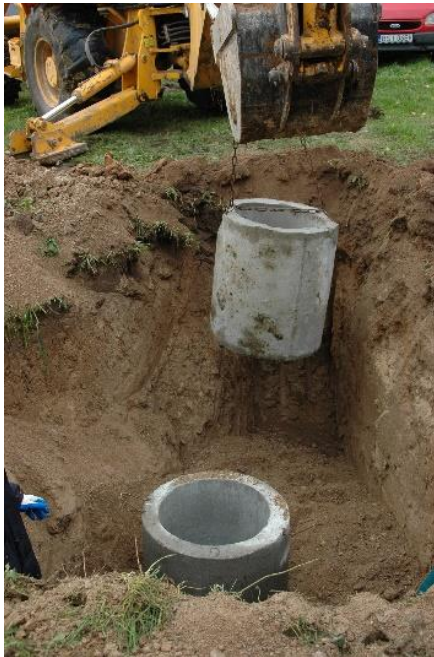
Figure 3. Installation of an absorbent well
