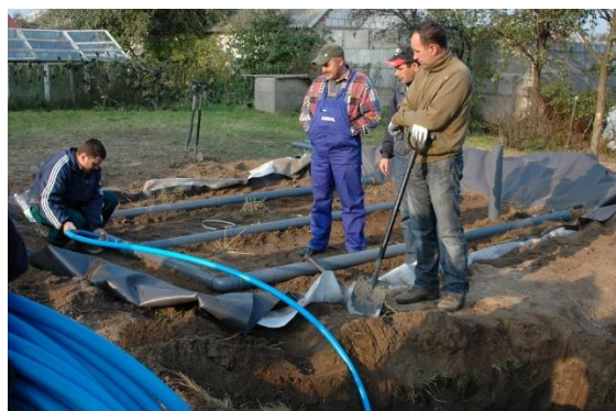
Figure 1. Connection of the settler tank to the infiltrating drainage
