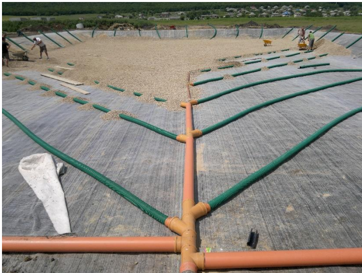
Figure 9. Backfilling the collecting drain with aggregate
