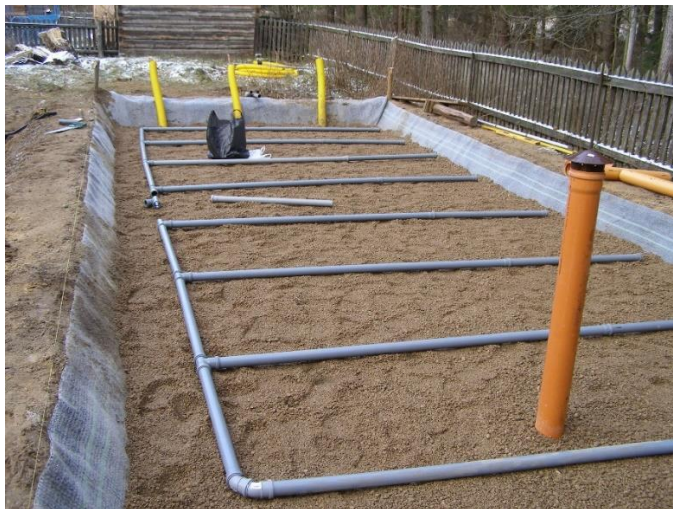
Figure 11. Laying out infiltrating drainage
