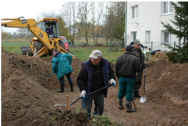
Figure 2. Excavation for a sand filter
